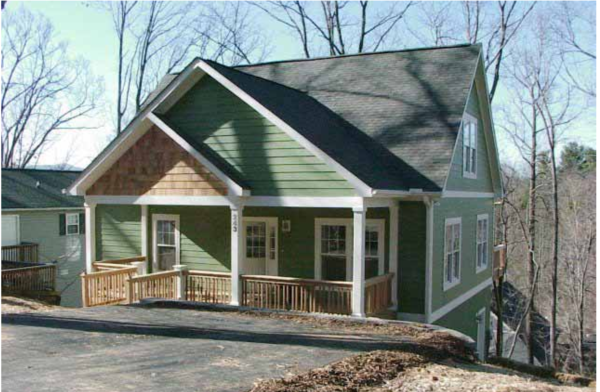
Innova Project1 on Westover Alley, Asheville, NC
