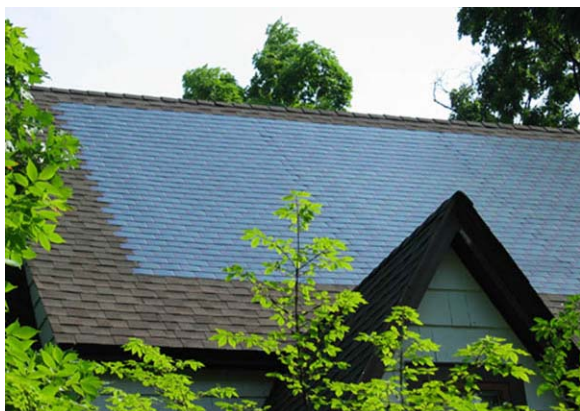
Figure 5. Amorphous Thin Film PV Shingle System
