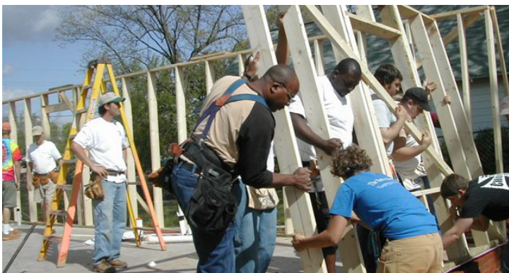
Figure 1: Habitat for Humanity framing crew at work
