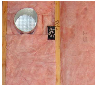
Figure 13: Proper insulation installation
