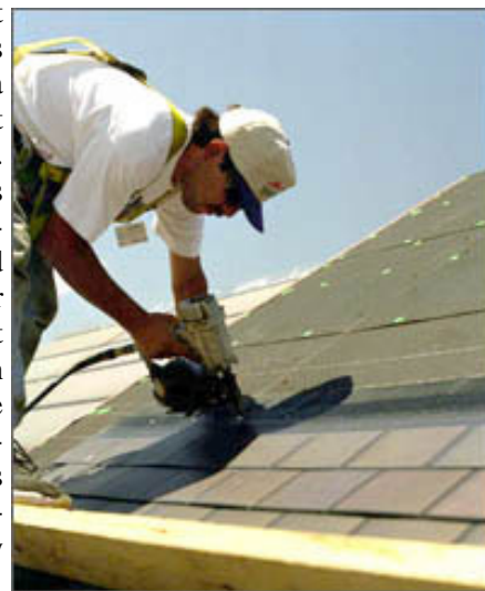
Figure 17: PV Shingle Installation
